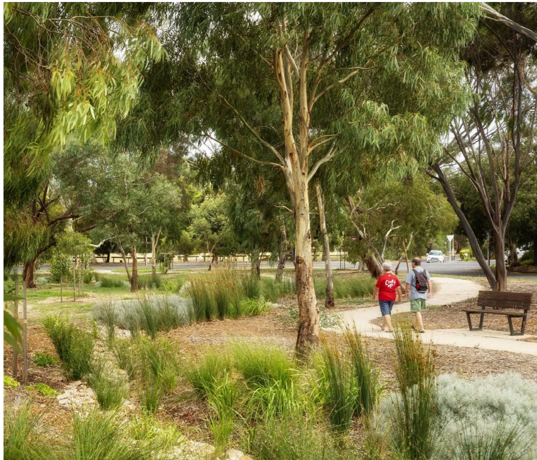
Vegetated detention basin
